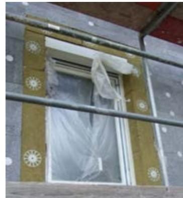
**Figure 26** : Plastic fasteners for insulation [Source PHI]
