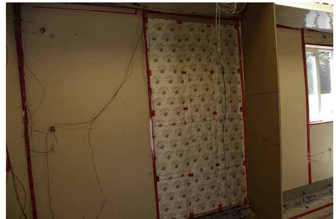
Fig. 2. PCM installation behind gypsum drywall.
