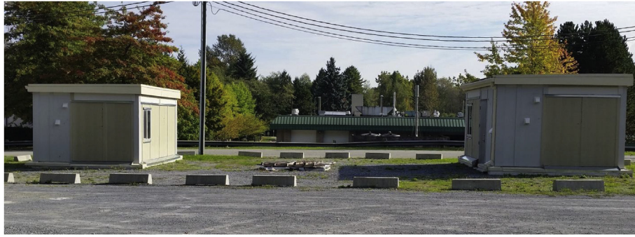
Fig. 1. From left: North (with PCM) and South (without PCM) Test Building.
